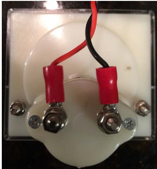
Figure 5.113 – Ring Terminals Installed
