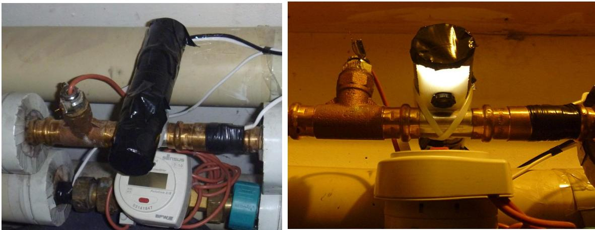
Camera in white plastic pipe. Leds also inside pipe.
