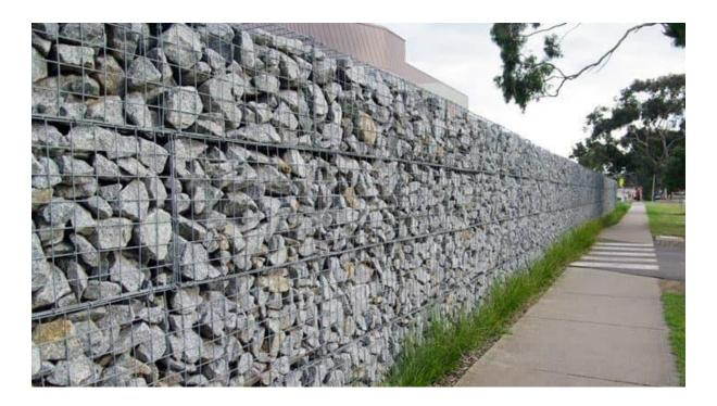
A series of wire cages hold rocks in place to form a really solid retaining wall or fence.
