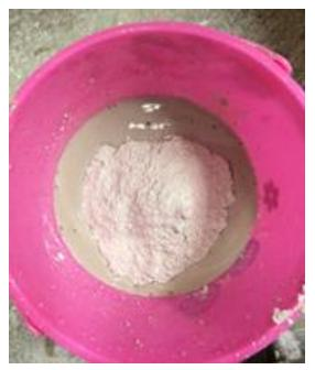
2. Add the Ultracal by sprinkling it onto the surface of the water. It will sink to the bottom of the bucket. Add cement until you have a small island in the water.
