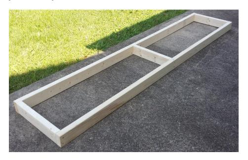
FYI, I almost forgot to measure the width of the doorway into the greenhouse and might have made the benches too wide. Luckily, my brain kicked in and I found that I had 22.25" to work with, so I planned on the benches being 22" wide overall. I cut some 2x4s down to 92" for the length per shelf and because a 2x4 is 1.5" thick and a 1x4 is 1.5" wide, I subtracted 6" from 22" and made the shorter 2x4 pieces 16" (you'll understand why later). I made all the 2x4 joints with 3" screws.
