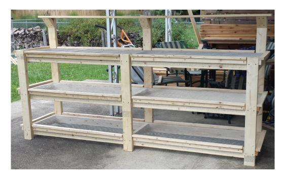
After moving the benches into the greenhouse, I realized the top 1x4 pieces on the ends of each shelf need to be removed because they interfere with the diagonal supports inside the greenhouse. I also needed to shorten the shelf a bit and I still needed to cut 4" holes in the wood to accommodate 4" flower pots.
