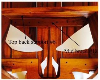
17-Install 3- 2" screws thru top back support and into mid back brace.
