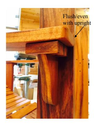
**9-**Predrill and install 2- 1 1/2" screws thru rear top plate of arm support and into the arm.
