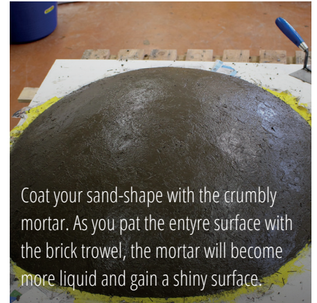
For the mortar you will need one part cement...
